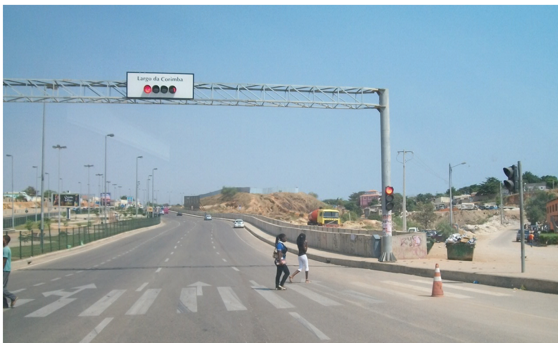
New road infrastructure in Luanda, Angola
